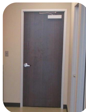
Opt 2. Office and Conference Rooms, Columbian Walnut Plastic Laminate Door with Brushed Aluminum Trim
