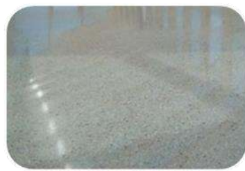
PS1 Polished Concrete Floors
